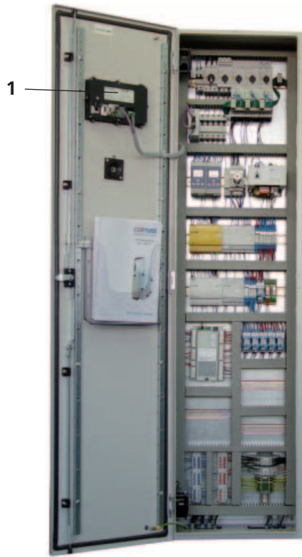
Schaltschrank Kombi Control cabinet combined version
